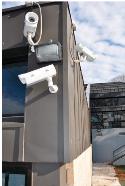
Five-megapixel cameras were situated to cover all angles, providing comprehensive surveillance for the school.
