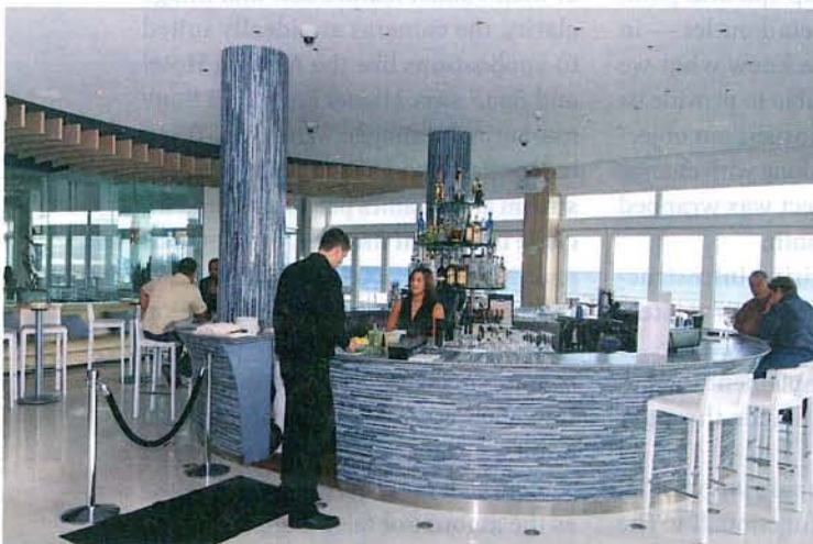
Sony dome cameras dot the ceiling of Allegria's scenic bar and restaurant. The new luxury retreat is located adjacent to the famous Long Beach boardwalk.
