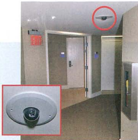
Hallway safety has been ensured via Sony DS-10 cameras featuring recessed mounting kits so as not to compromise the décor.
