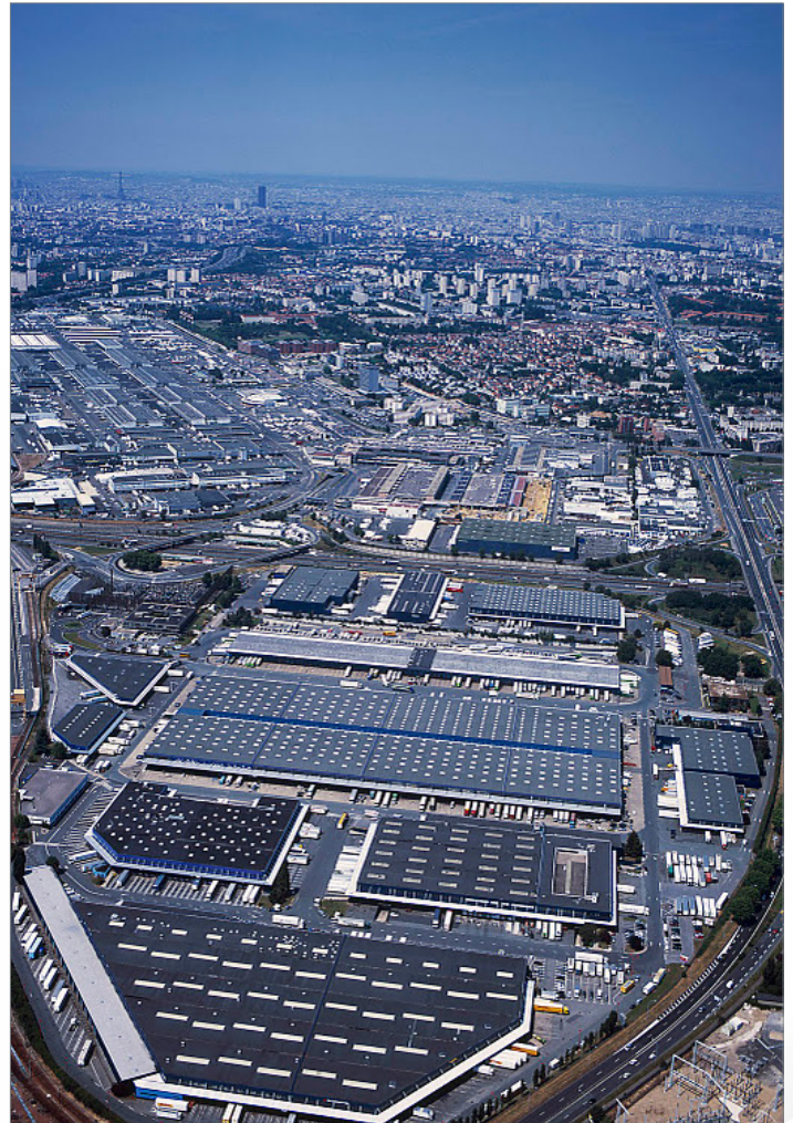
Arecont Vision's megapixel technology is now located throughout Sogaris, which currently manages seven logistic platforms with nearly 480,000 square meters of facilities.
