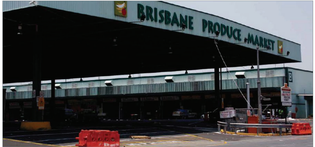
The Brisbane Markets Commercial Center is protected by a surveillance system using Arecont Vision MegaVideo® IP megapixel cameras.
