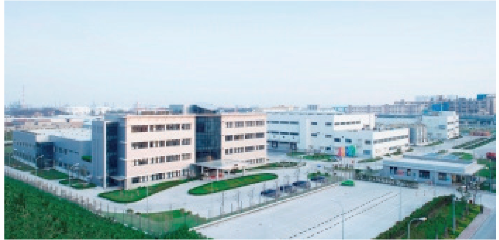
BASF China uses Arecont Vision dual sensor AV3135 IP megapixel cameras to provide video security 24-hours a day in normal and low-light conditions.
