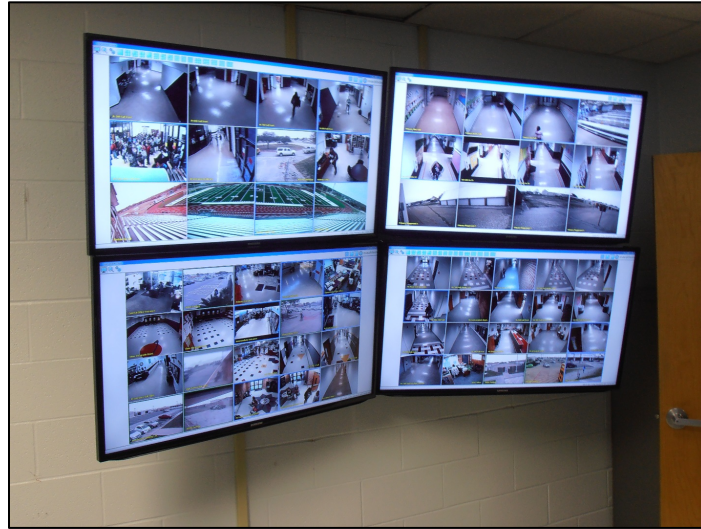
Monitoring station with 4 - 42" HDMI monitors running exacqVision software and video from the Arecont Vision® cameras
