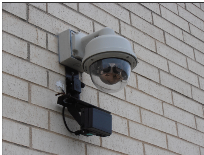
Arecont Vision® AV40185DN installed on auditorium with illuminator
