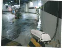
looking to improve the image clarity provided by security cameras watching parking entrances. He explained that the store receives claims of damage to cars while parked in the store's lots. The previous system used cameras that provided resolution inadequate to supply a clear view of the exterior of cars entering the parking area. Lotte wanted to be able to confirm whether a car already had damage as it entered the parking lot.
